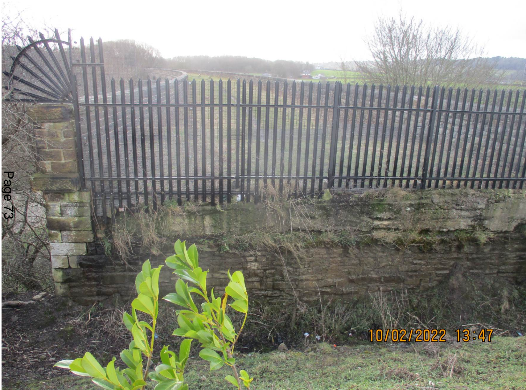
Photo 2 – Photo taken by Council Enforcement Officer February 2022 (post engineering works)
